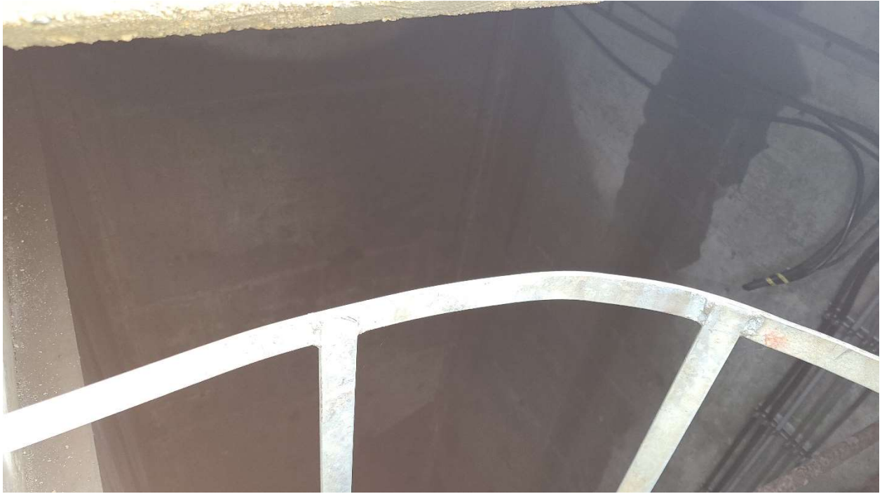
Photograph #21: LAV-1 Valve Pit
