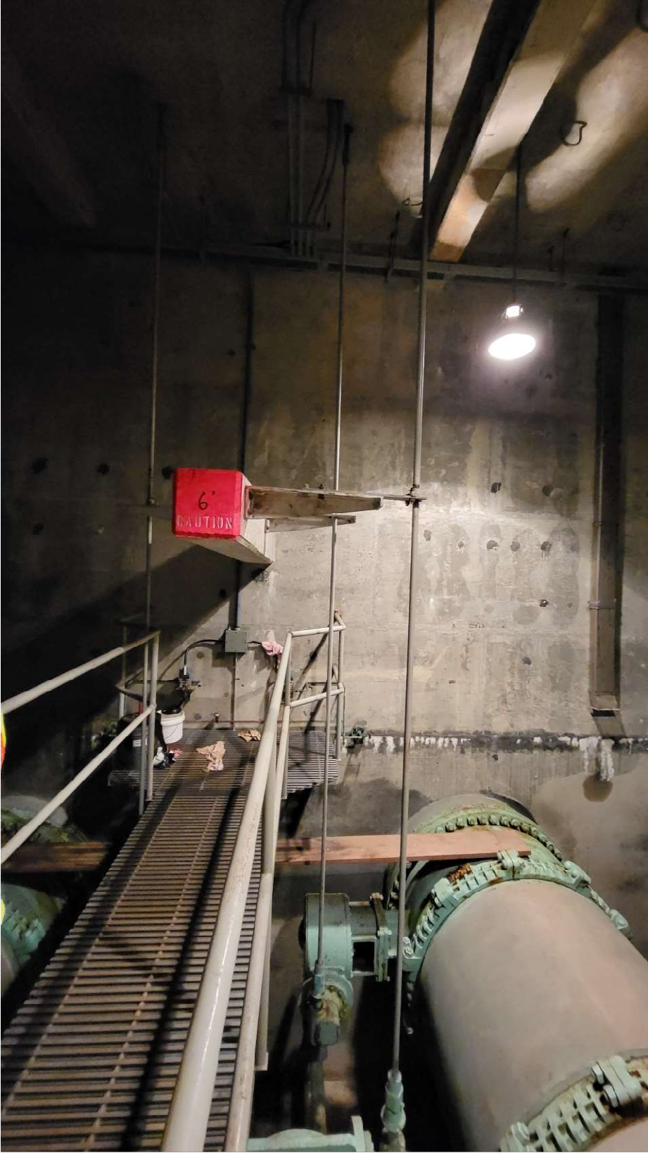
Photograph #12: Valve House Pit
