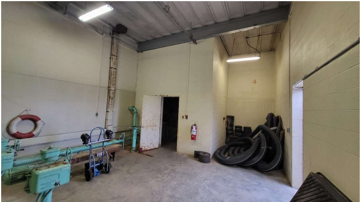
Photograph #18: Valve House
