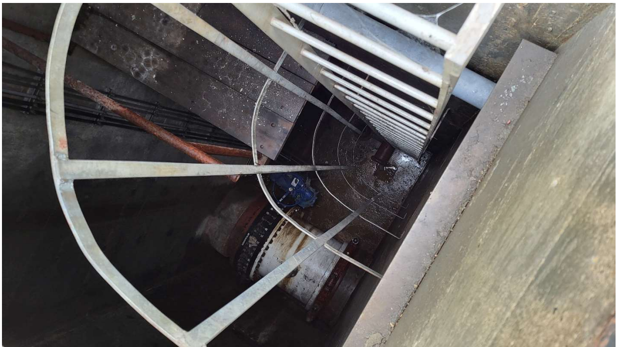
Photograph #22: LAV-1 Valve Pit
