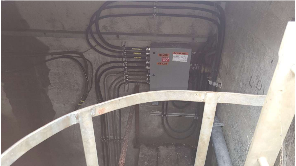
Photograph #19: LAV-1 Valve Pit
