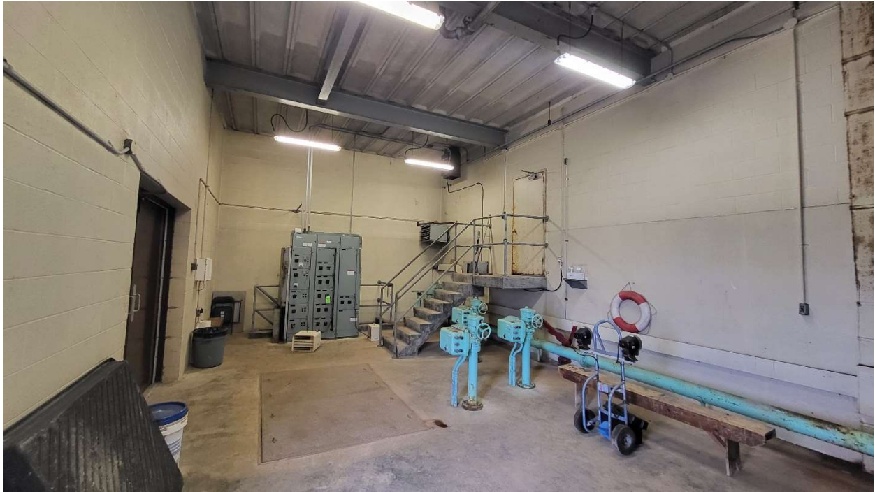
Photograph #17: Valve House
