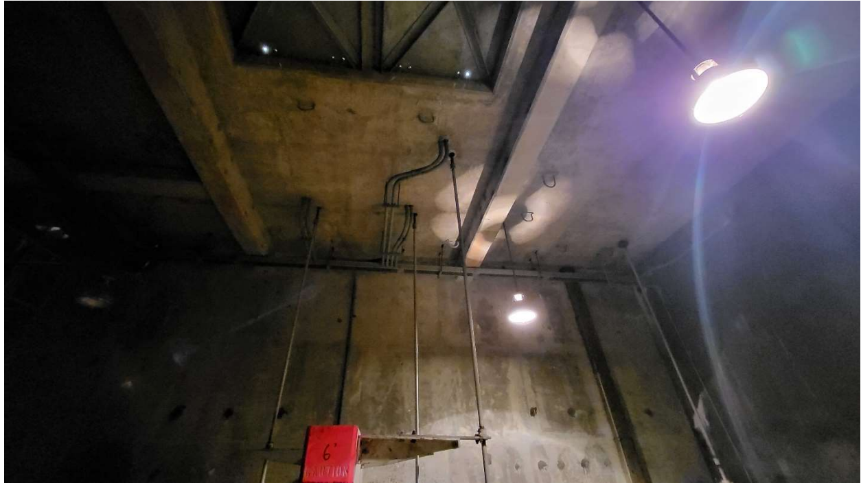
Photograph #10: Valve House Pit
